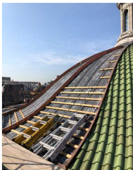
Ludowici terra cotta tile roof replacement in progress.
