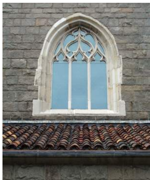
Restored limestone window and roof tiles, new protective glazing.
