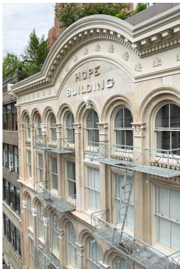
Restored street facade.
