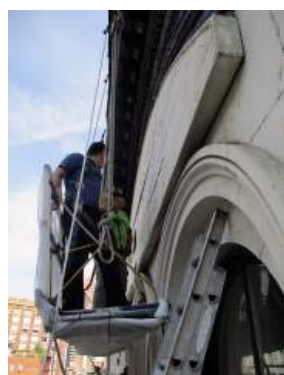
Covered signage and damaged cornice, pre-restoration.
