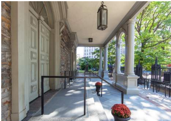
Permanent accessible entry ramp and restored portico.
