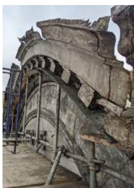
Covered signage and damaged cornice, pre-restoration.
