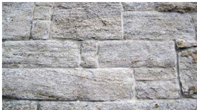
Tan-gray sienite stone of the exterior walls.
