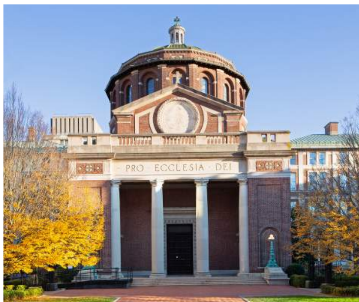
Restored brick and limestone main facade. Photograph by Bilyana Dimitrova.
